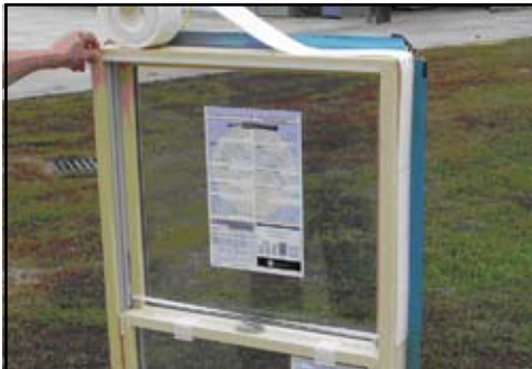
Figure 2 – A non-biodegradable material treated with a diffusible preservative can be applied to pre-hung windows at the factory, building site prior to installation, or in place on existing windows.
