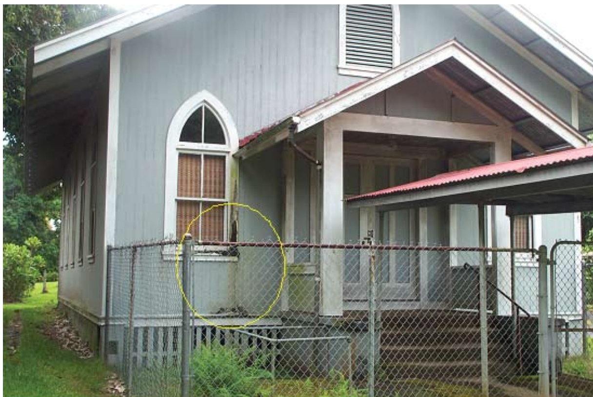
Figure 1 – Wind-driven rain and/or building design features that direct moisture to windows are some of the many ways moisture penetrates wall openings.
