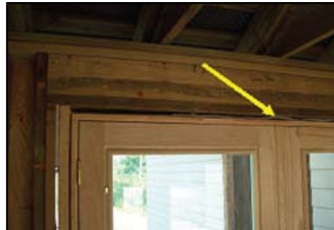
Figure 3 - A non-biodegradable material treated with a water - diffusible preservative can be applied to pre-hung doors at the factory, at the building site prior to installation, or while in place.
