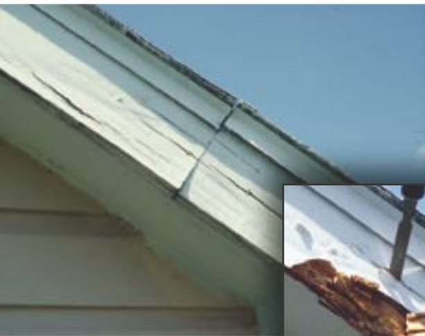
This fascia board was exposed to rain water which soaked in the board ends. Note the cracked appearance of painted wood and the brown, soft wood in the inset.
